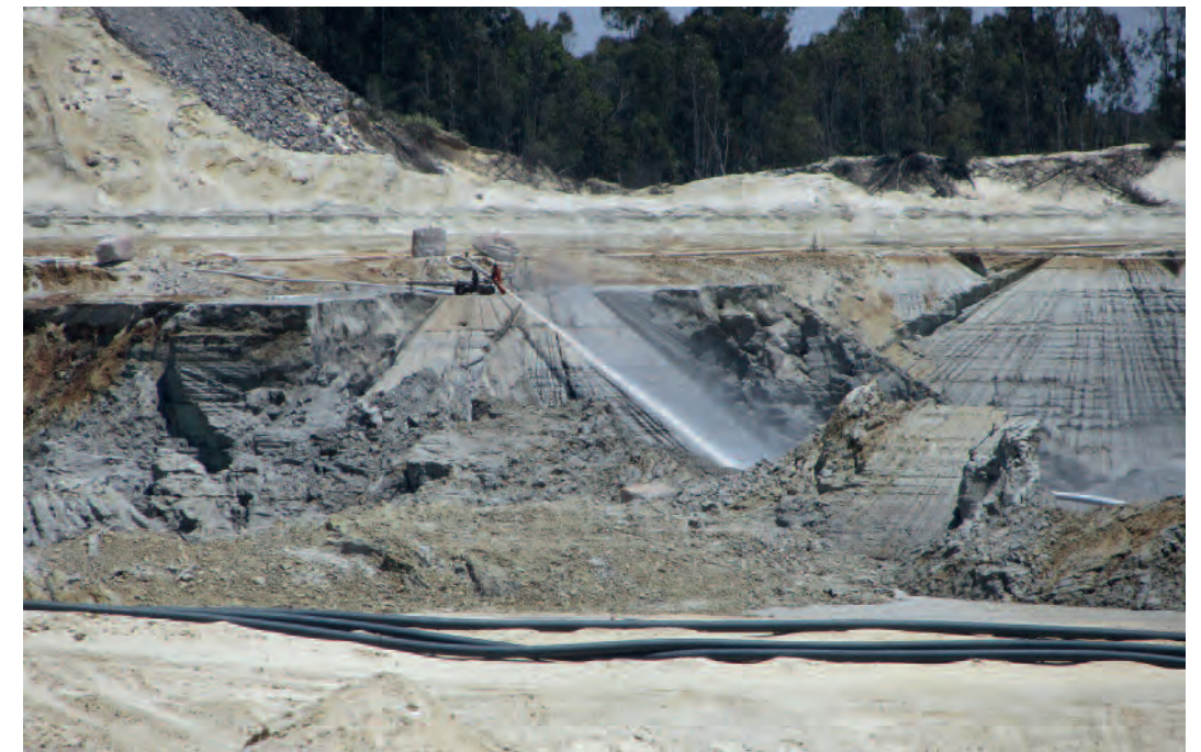
Remining can generate AMD because it uses water cannons to process the tailings, as shown here at the Sand Dump No. 20 reclamation site. © 2014 Bonnie Docherty/IHRC.
