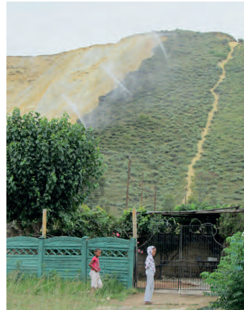
Sprinklers and vegetation helped control dust at this tailings dam next to Riverlea in the Central Rand, but they did not eliminate the problem. The government has not ensured the systematic and effective use of such measures in the region. © 2012 Bonnie Docherty/IHRC.
