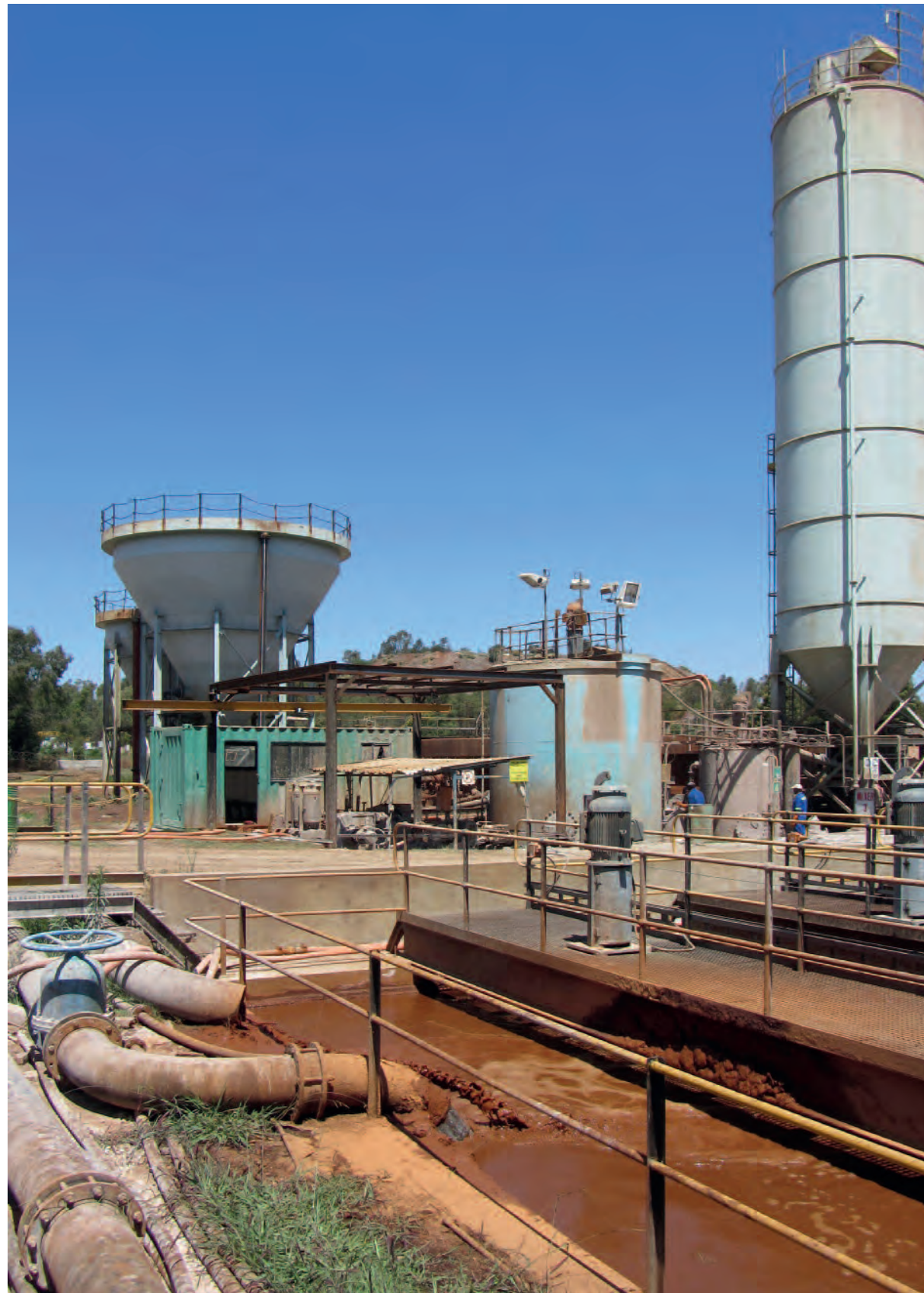
AMD finally stopped decanting after the government assumed responsibility for the West Rand Treatment Plant and increased its capacity. While a critical short-term fix, the plant has only neutralized the water and has sometimes been overwhelmed by heavy rain. © 2014 Bonnie Docherty/IHRC.
