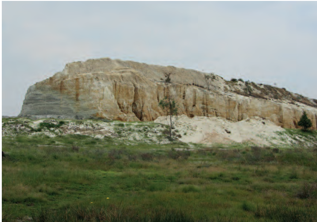
This large tailings dam, which was being remined in 2014, was situated near the Afrikaner community of Mindalore in the West Rand. © 2014 Bonnie Docherty/IHRC.
