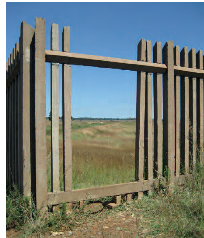
Large gaps in the fence surrounding Donaldson Dam have given Bekkersdal residents easy access to the contaminated body of water. Local people have stolen the concrete-covered rebar to sell for scrap metal, and the government has not adopted a better solution to cordoning off the dam. © 2010 Bonnie Docherty/IHRC.
