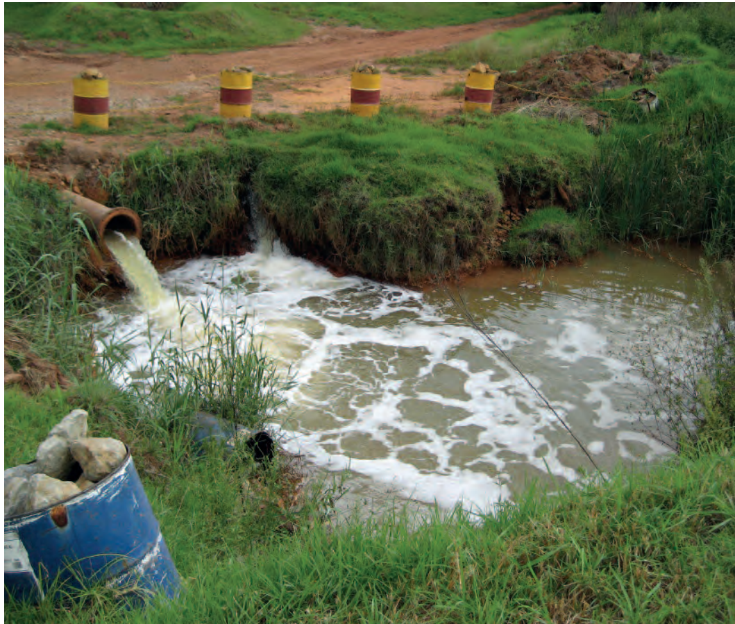
In 2010, a pipe released decanting AMD into a culvert that flowed directly into the Krugersdorp Game Reserve, endangering wildlife. Since then, the water here has reportedly been treated, but the sulfate levels have remained unacceptable. © 2010 Bonnie Docherty/IHRC.
