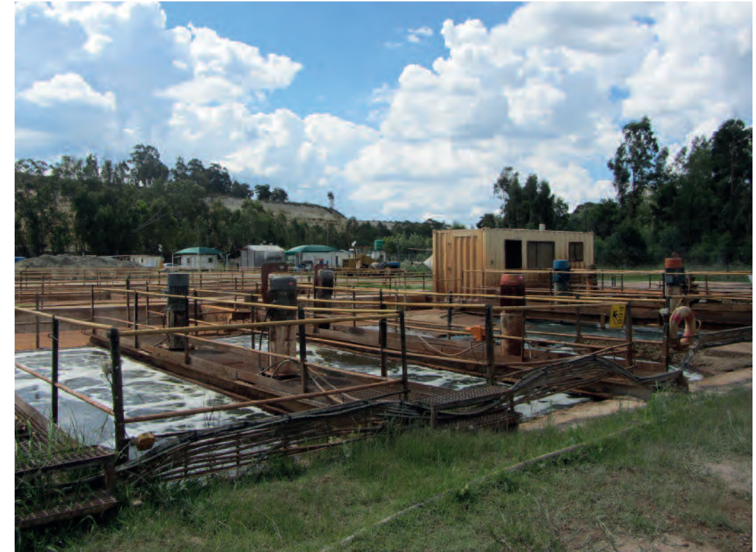
Industry led early efforts to stem and treat decanting AMD in the West Rand. This facility operated by a mining company helped address the crisis but could not handle the large quantities of contaminated water. © 2012 Bonnie Docherty/IHRC.
