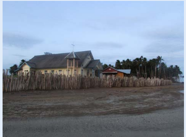
The church behind its sea wall
