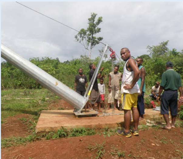
Raising the wind turbine pole at Bishop Koete RTC.
