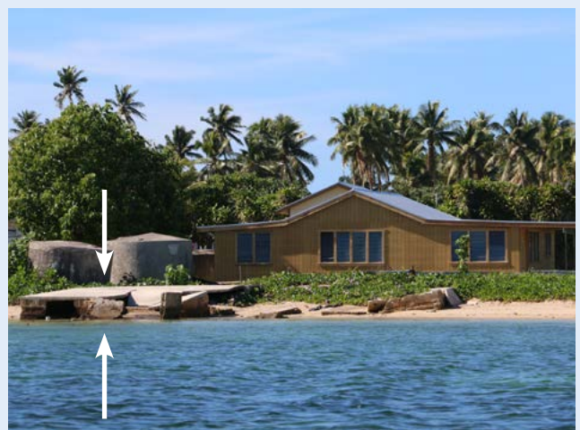
May 2017: Foundations only
