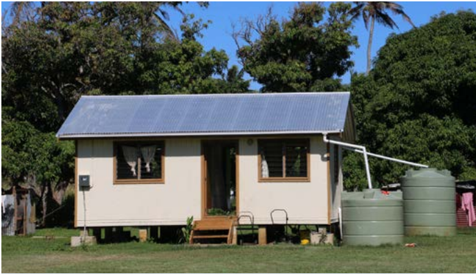
This new house in Ha'apai has been built using cyclone-resistant materials and techniques.
