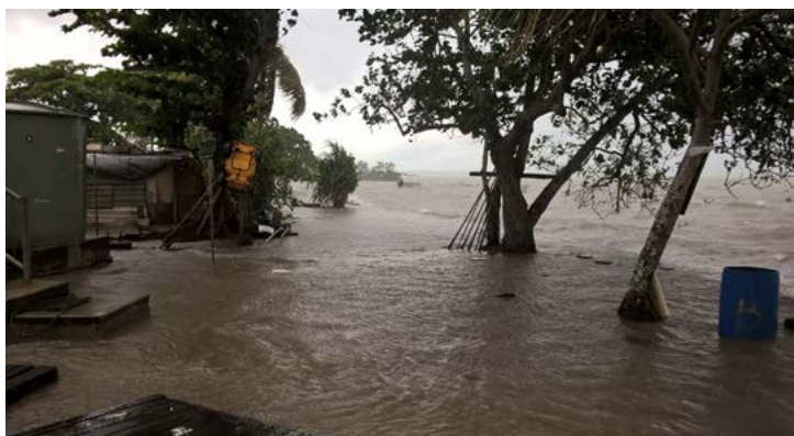
Flooding at Boigu, Torres St Islands, Australia February 2017.
